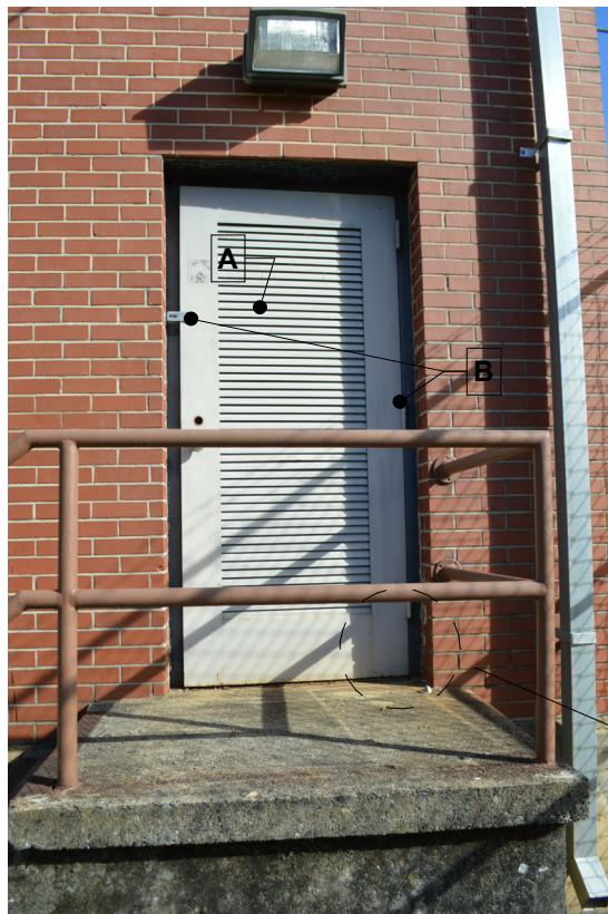
SWAT BUILDING OUTSIDE STORAGE ENTRANCE DOOR
