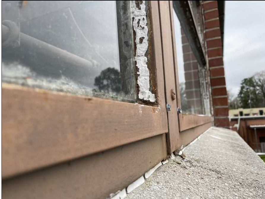
3 - View of ACM window glazing and caulking.
