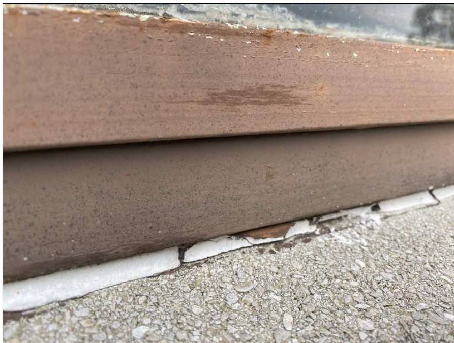
2 - Additional view of ACM window caulking.
